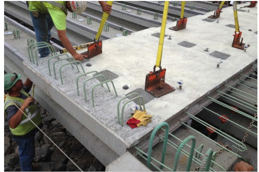
Precast Deck Panel Installation
